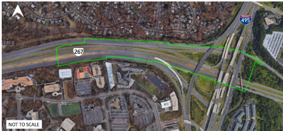
Figure 8-9. Route 267 Interchange Zone: I-495 (Dulles Toll Road Mainline Only)
